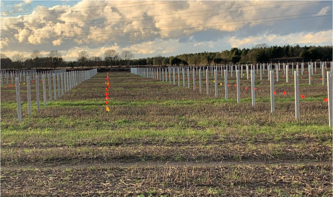
Insert 31: Legs Being Installed January 2023
